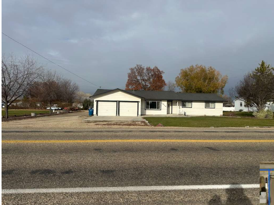
Figure 1 Facing north on E Victory from the western driveway
