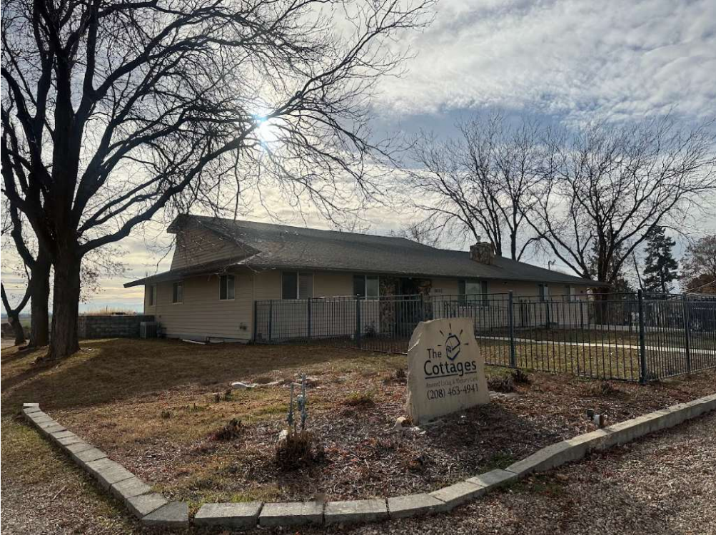
Figure 11 Facing southwest on E Victory from the eastern driveway
