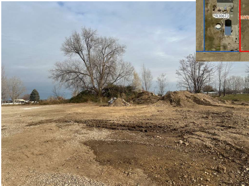
Figure 18 Facing east from proposed staging area location
