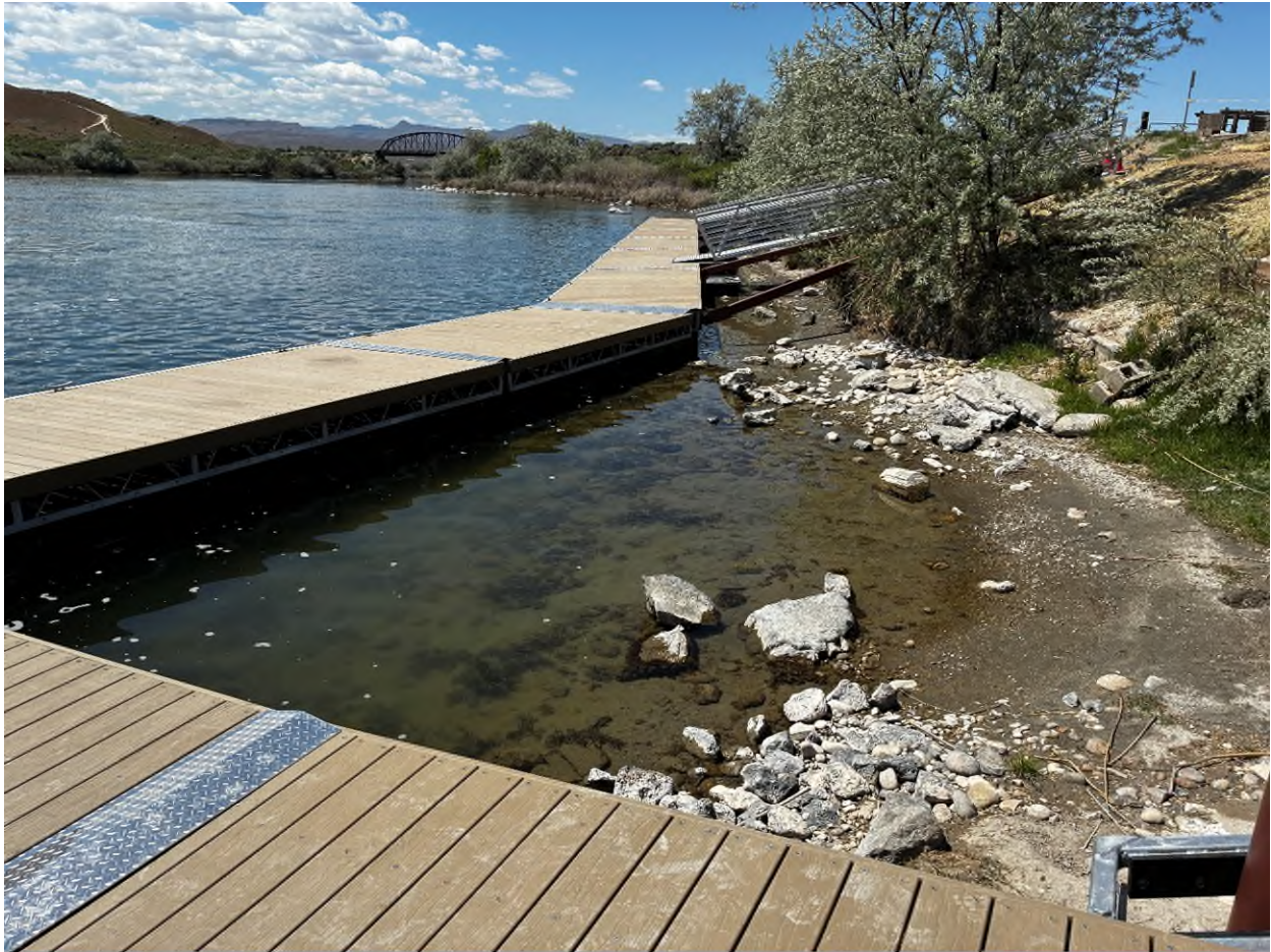
New docks and west gangway.
