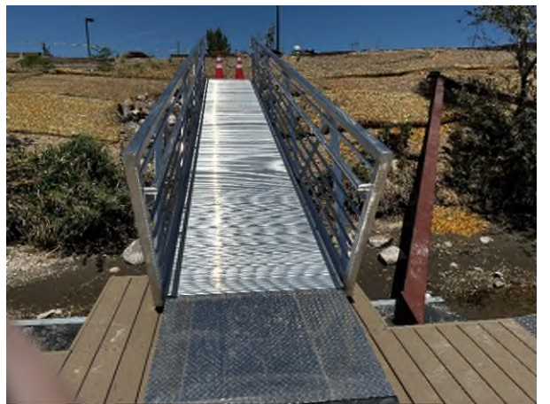
After: West gangway.
