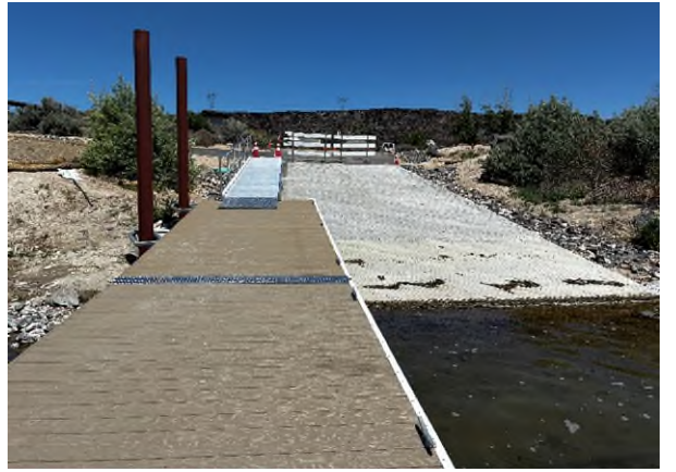
After: East main gangway.
