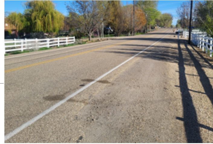
Pit Lane Facing North
