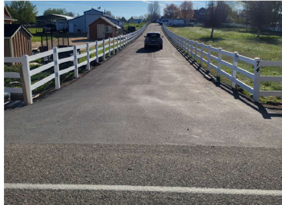
Paved Driveway Entrance to Pit Lane
