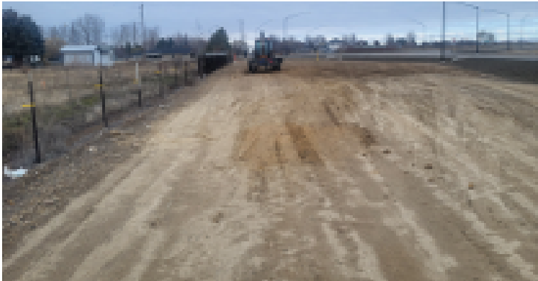
Facing North on Public ROW Dedication along Eastern Boundary of Property
