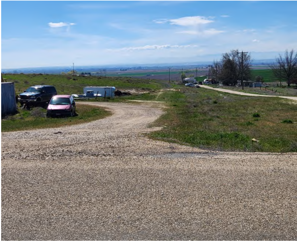
The proposed private road to serve the properties runs parallel approximately 40 feet from edge of the adjacent driveway to the west. As proposed the access would serve three properties requiring a private road lot for the purpose of platting.
