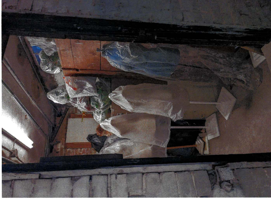
Nampa Depot Museum Dehumidifier Grant Request Basement Photo 1
